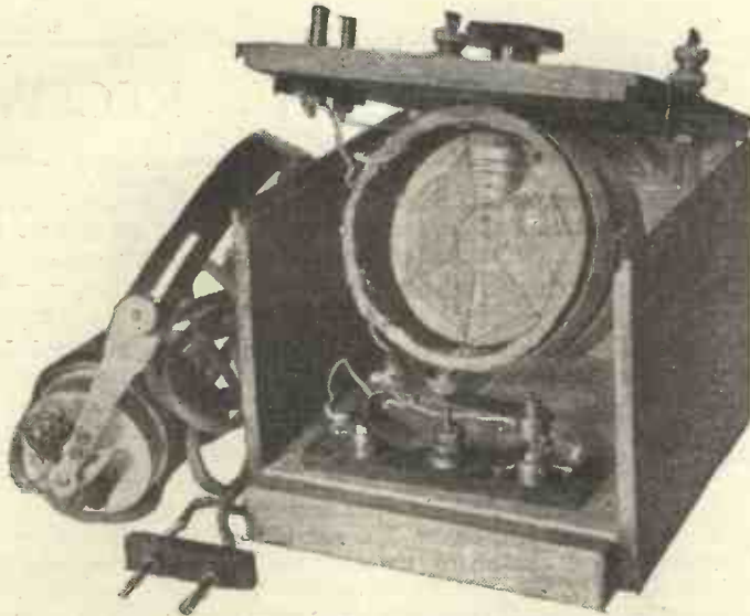
Fig. 2.—The box open, showing simple variometer.
